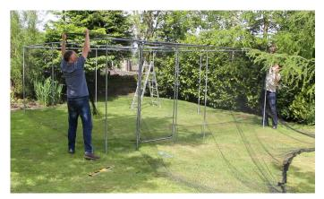
Pull top net over the whole cage, ensure equal amounts to each side.
