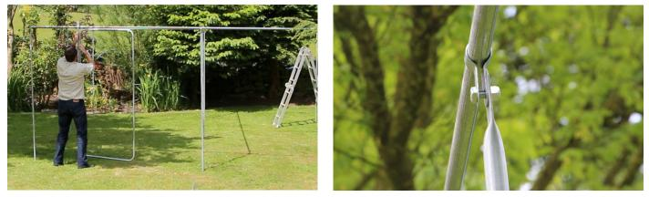
Push door post into ground, and secure to keyhole bracket (using two 17mm spanners) as shown above.
