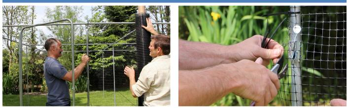
Start at the right hand door post, secure netting with cable ties (approx. one at top and a further four on the post). Cut net around the door latch.
