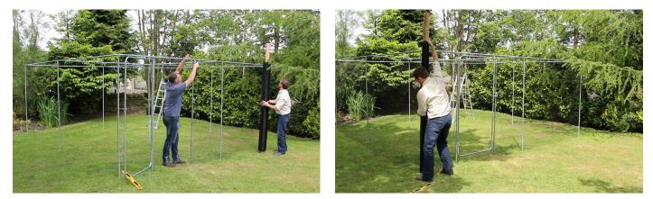
Roll out the netting around the cage, ensure you pull it tight and secure with cable ties as you go.
