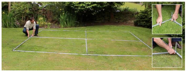
Lay out the roof components on the ground as shown (each style of fruit cage is different so this will ensure you have the overall shape correct). This layout can then be used as a guide for the upright posts.
