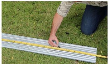
To assist in achieving the correct height, lay out the fruit cage posts (ensuring the are in-line), then using a tape measure mark at 1.9m.
