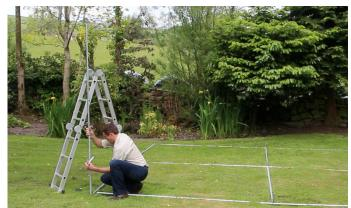
Detach one of the corner fittings. Place the upright in its place. Re-fit the fitting to the top of the post.
