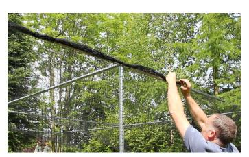
Roll-up any excess net and secure with cable ties.
