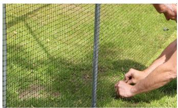
Finally secure at the base with ground pegs, approx. 2 per 2.5m section.
