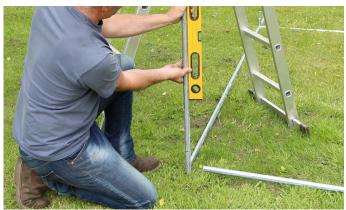
Check the post is level as it is going in. Continue until the mark you made is at ground level.
