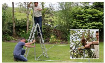
Use a wooden block and mallet to drive the tube into the ground.
