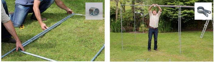
Slide one door post (with flattened end at top) through the first door hinge and add one hinge collar, continue to next hinge and add another collar then loosely tighten. At the point you wish to fix the door, clip keyhole brackets to frame.
