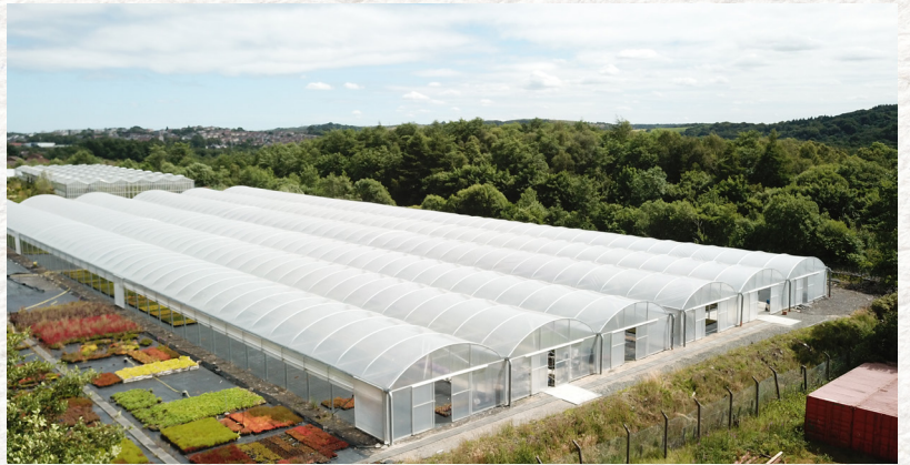
48m Wide x 75m Long Multi-Span Polytunnel
