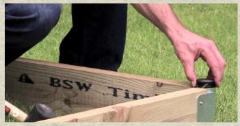
Raised beds with side brackets are supplied with support rods. These slot in to the small corner gap between the inside back plate and the tube part of the side bracket (4). The support rods will prevent the sides of the raised bed bellying out. Insert the protective plastic caps on all of the brackets (5). This is easier done with a mallet. These can be prized out at a later date if you decide to extend the height of the raised bed, or if you add one of our raised bed hoop kits.
