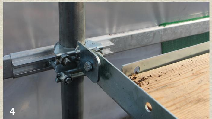
You should now have a study frame, with 4 sides and 2 central support bars. Using the fittings provided secure the frame to your polytunnel hoops. Be careful not to over-tighten the bolt that connects the bench to hoop, as this will act as a hinge allowing the bench to be folded away.
